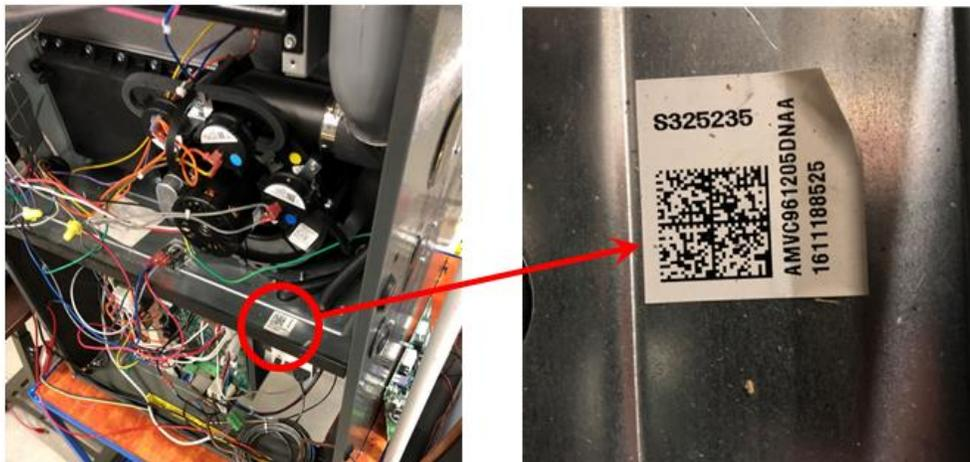
*For this **ComfortNet™** furnace, the 2D barcode is located on the blower deck, its model number is AMVC961205DNAA*
