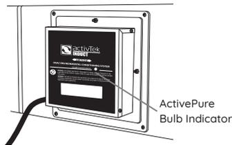
8. Re-install unit if removed from duct. Reconnect power and check for proper operation.
