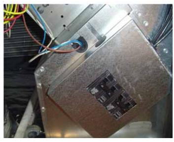
**FIGURE 9**16. Install control box door and blower door.
